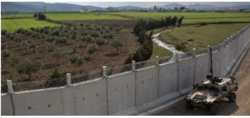
PROTECTION WALL OF PCC
